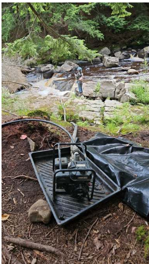
Pump supplying water to drilling operations only hundreds of feet from the Huron River.
