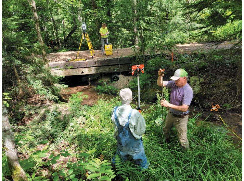
Deer Creek data collection 2022: Olivia Engelhart of GEI (on bridge) with John Highlen and Doug Vanerka of TU preparing to take a depth of refusal measurement, which determines the amount of sediment buildup on the original streambed. Photo by Mitch Koetje.
