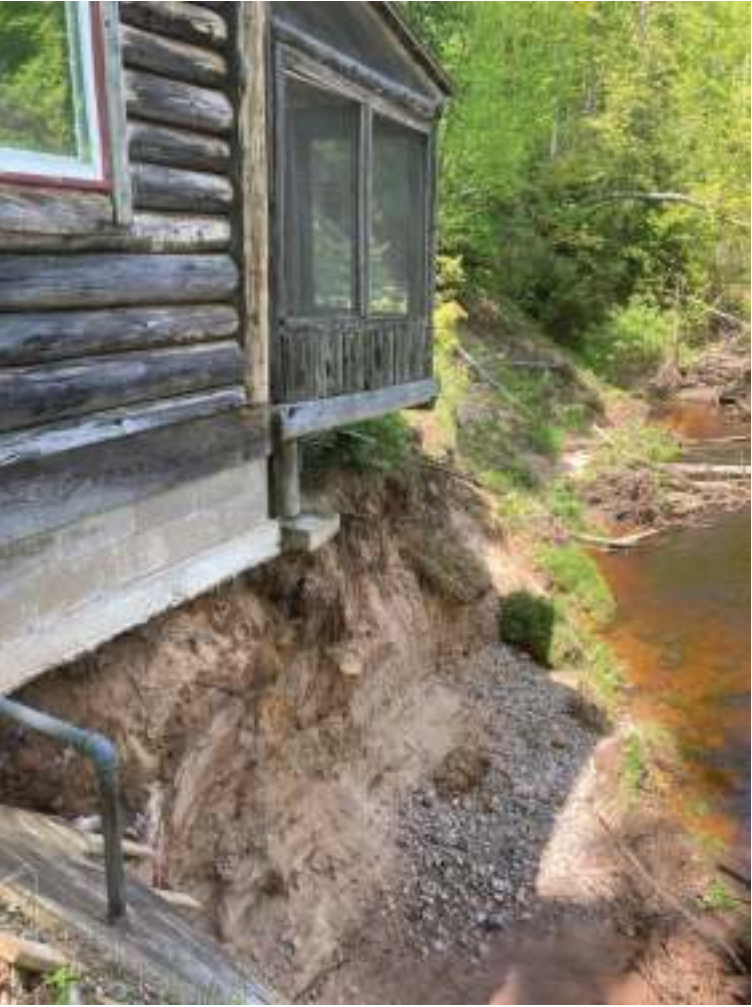
A cabin constructed too close to the Yellow Dog is now in danger of collapsing into the river. When it was built, this structure complied with Ishpeming’s present setback regulation of 30 feet. Photo by Kristi Mills.
