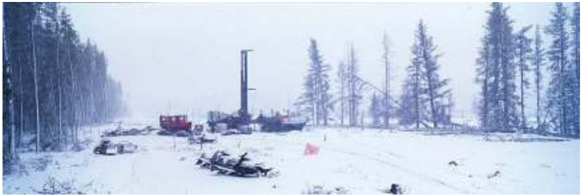
Top panoramic: In the winter of 2004, Ted captured this panoramic image of a rig drilling a water-monitoring well not far from the future site of Eagle Mine on the Yellow Dog Plains. Ted had hitched his snow cat (the orange machine to the left) to a drag and hauled water to lubricate the rig’s drill bits, a 2-hour one-way trip from operation headquarters in Big Bay.
