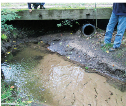
Deer Creek crossing. Water is forced to flow underground, beneath the bridge, due to culvert failure. Photos by Jan Zender.
