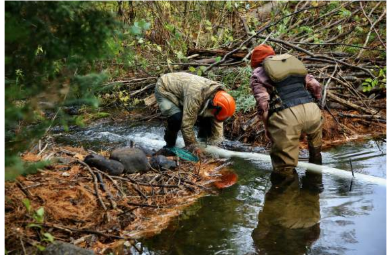
Chauncey Moran and Jacklyn Lenten installing a water pipe through a beaver dam to facilitate water drainage. Photo by Nancy Moran.
