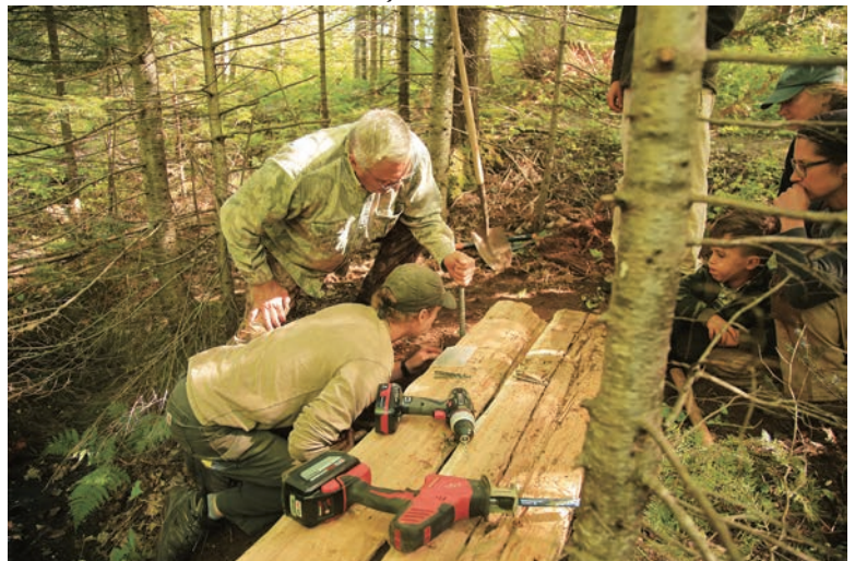
John Anderson with Abraham Turner: setting rebar to secure foot bridge. Photo by Chauncey Moran.
